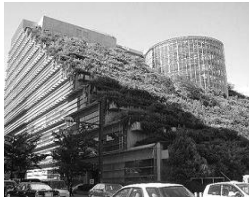
Green projects, such as those involving green roofs, will receive special financing through the Green Project Reserve in the 2010 financial cycle.
