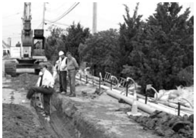
Sewer line construction in Brick Township.
